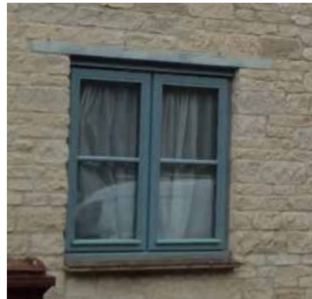
Casement window flush with wall, Bletchingdon
