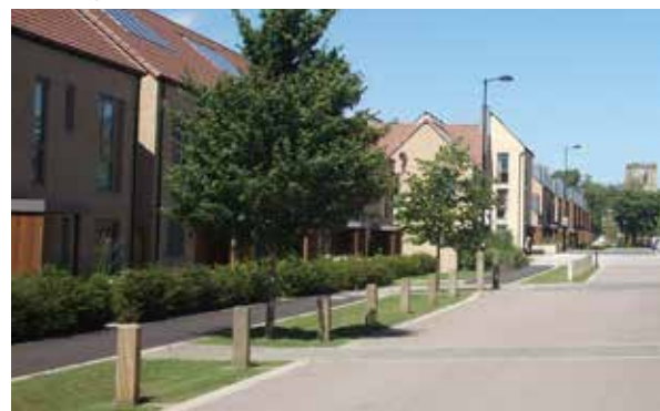
Incorporating SuDS along kerbside, Trumpington Meadows, Cambridge
