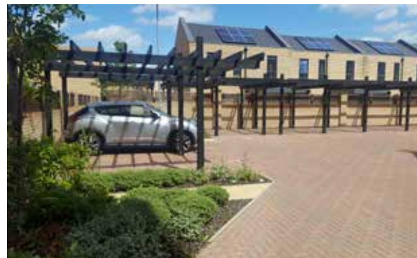
Well landscaped rear court parking, Clay Farm, Cambridge
