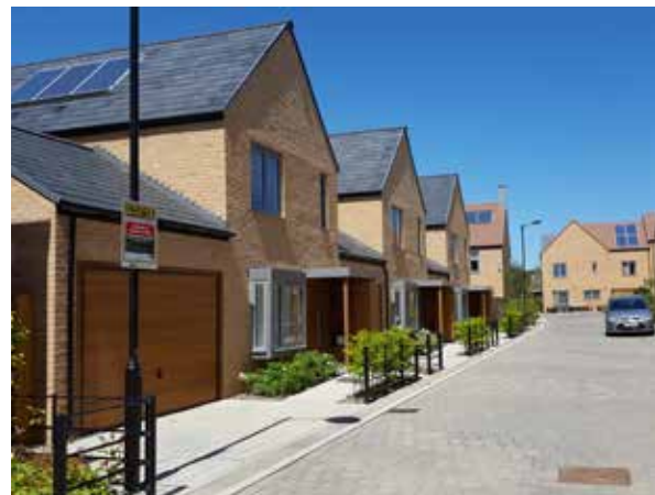
Photovoltaic panels, Trumpington Meadows, Cambridge
