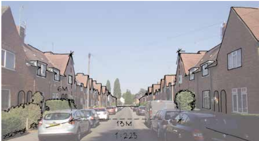
c) Queens Road, Banbury
