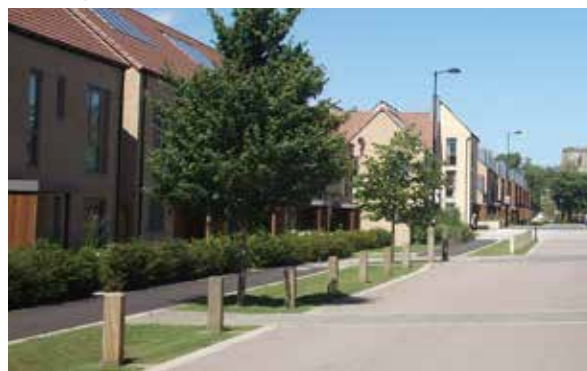
Incorporating SuDS along kerbside, Trumpington Meadows, Cambridge
