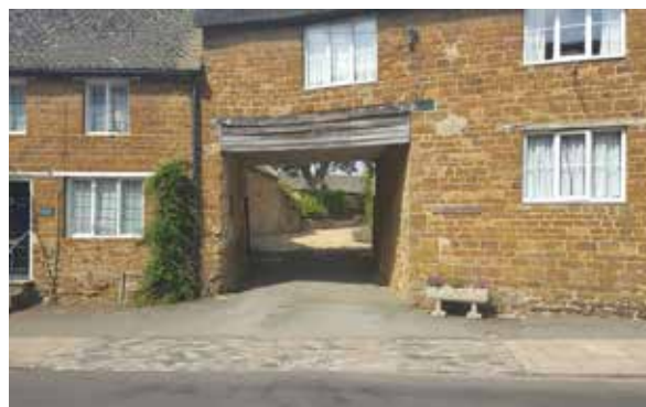
Rear parking accessed through carriage arch, High Street, Adderbury
