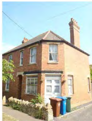
Cutting off edge to address corner, Islip
