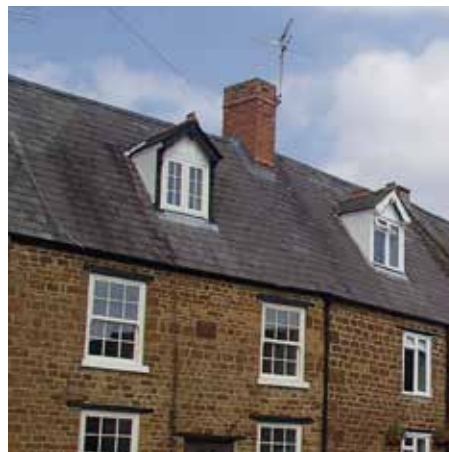
Rectangular brick chimney at edge of mid-terrace dwelling, central to gable, Adderbury
