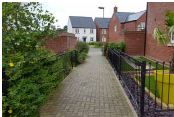
Pedestrian/ cycle cut-through, South West Bicester
