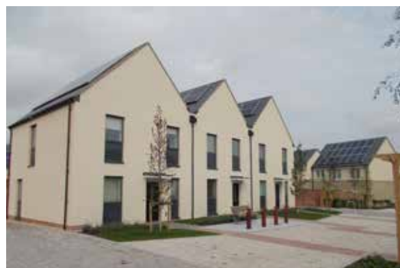
A shared surface street - NW Bicester
